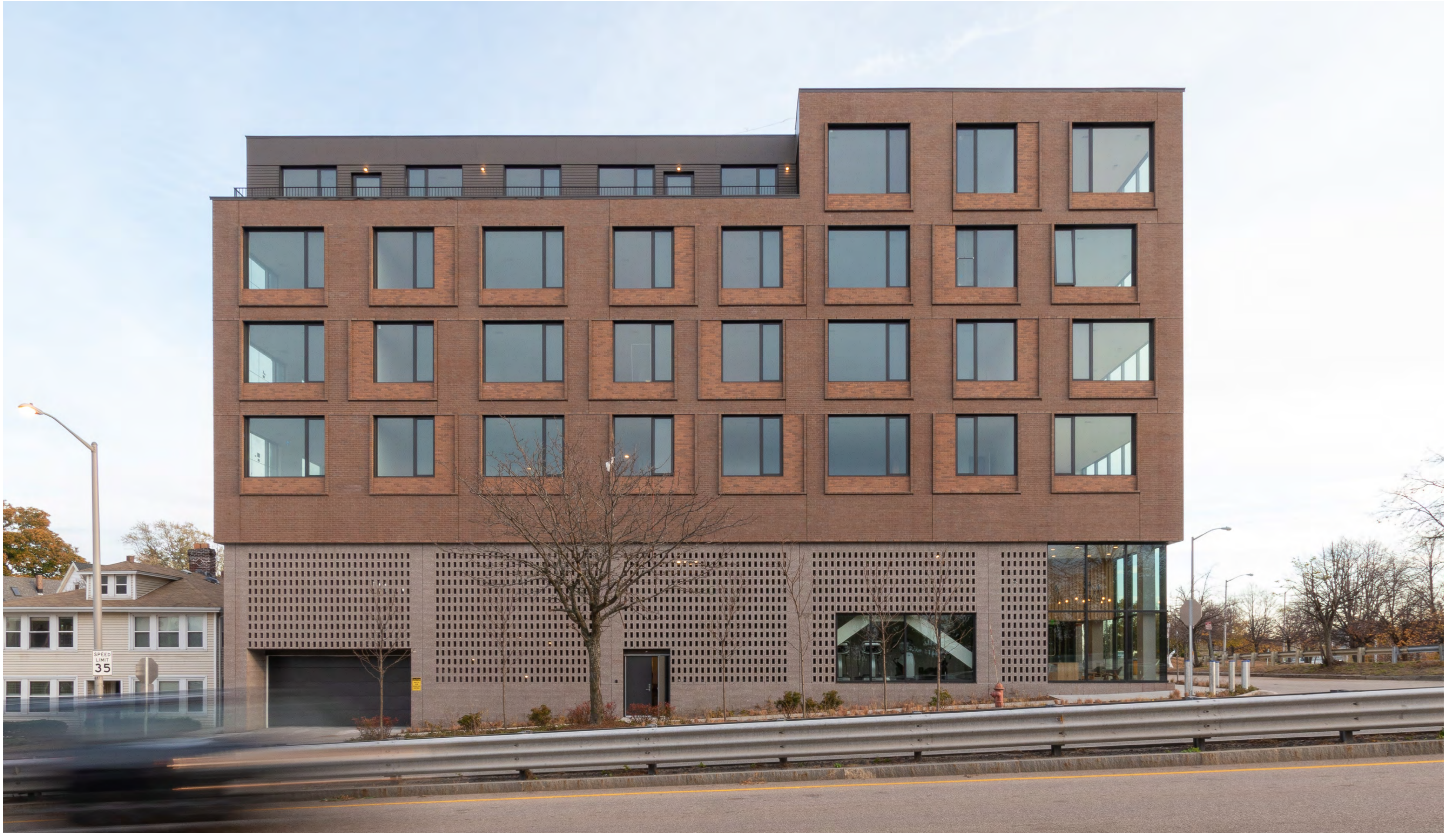
Oversized windows within an array of large brick apertures give movement to the facade while also scaling down the overall reading of the massing
